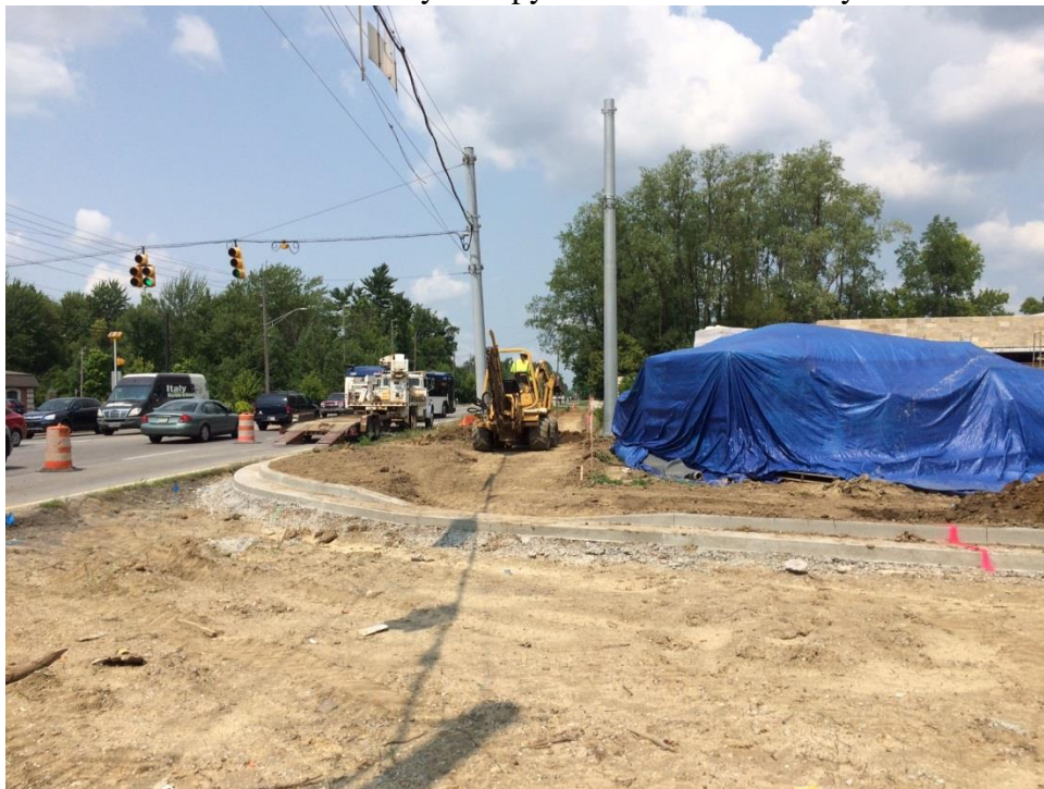
Project Site on August 14, 2018 View of the new sidewalks along Michigan Road.
