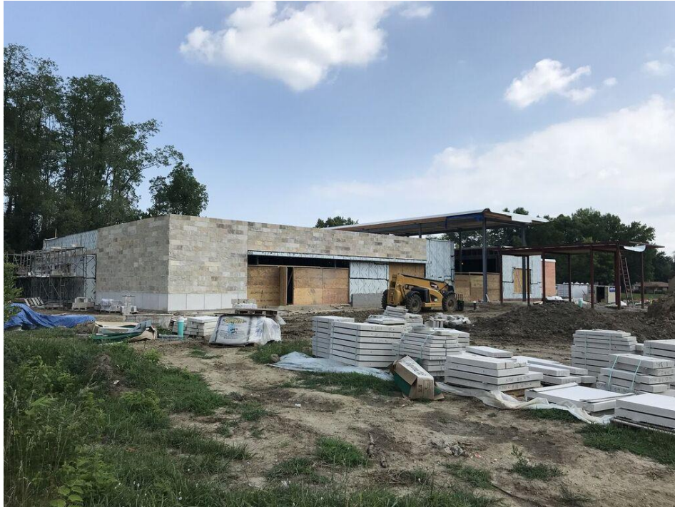
Project Site on August 1, 2018
