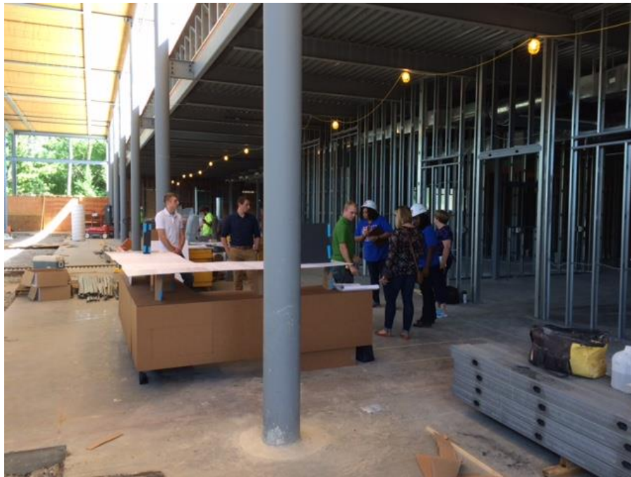
Project Site on July 25, 2018
