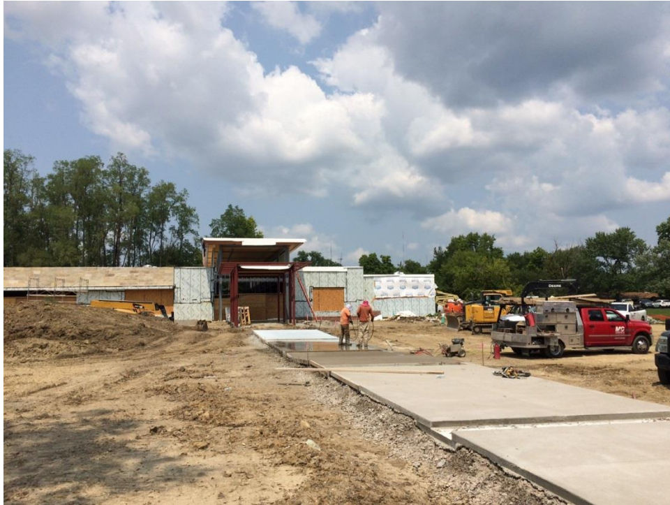
Project Site on August 14, 2018 View of the entry canopy and the new walkway.
