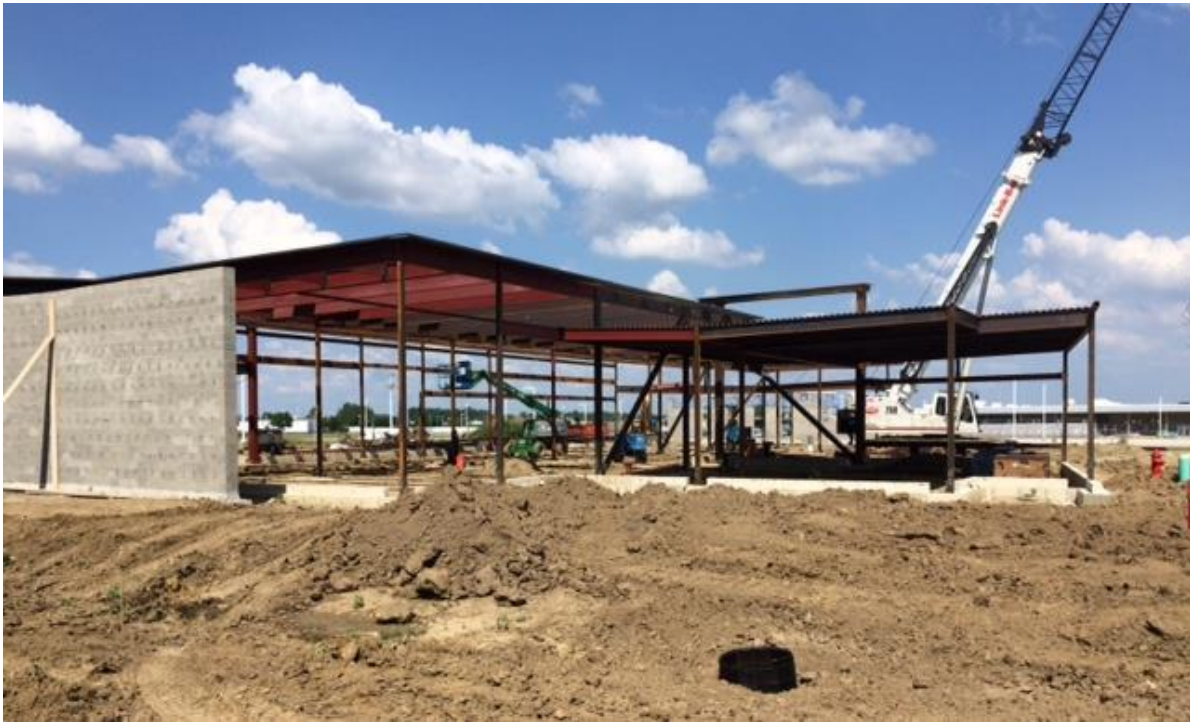
Project Site on July 25, 2018
