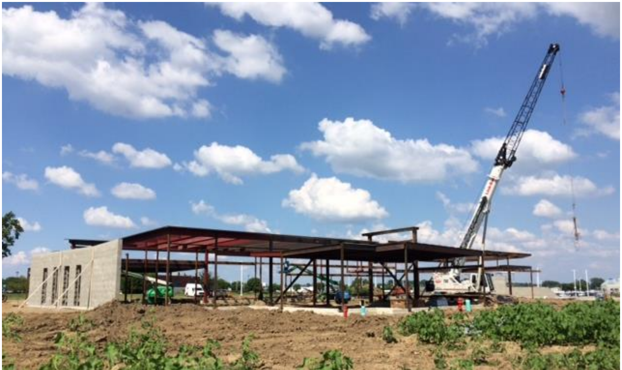
Project Site on July 25, 2018 View from Moller Road with steel installation in progress.
