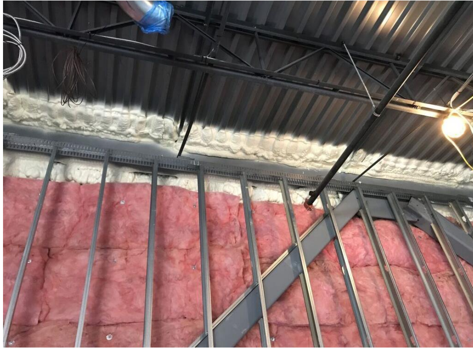
Project Site on August 1, 2018
