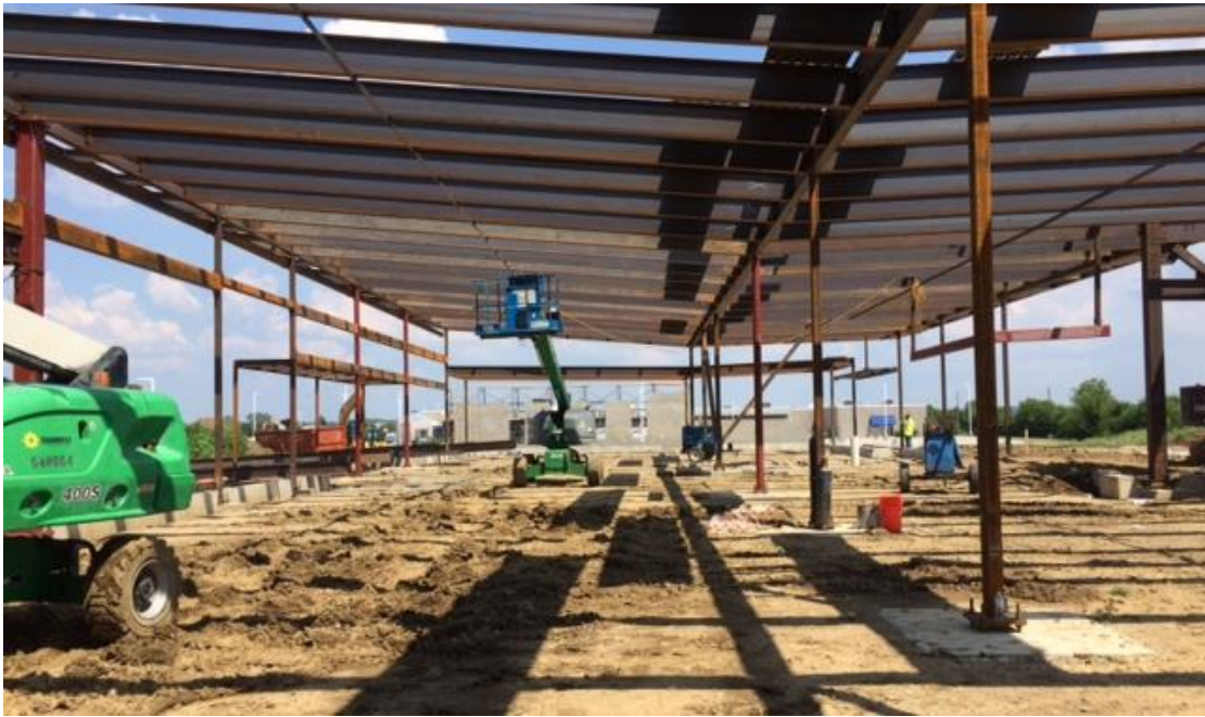
Project Site on July 25, 2018
