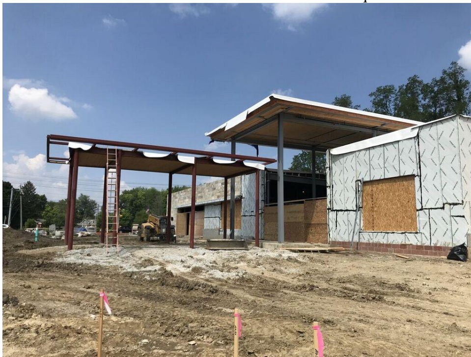
Project Site on August 1, 2018
